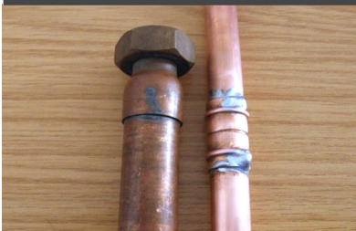
22mm pipe with lead solder and 15mm pipe with lead free solder
